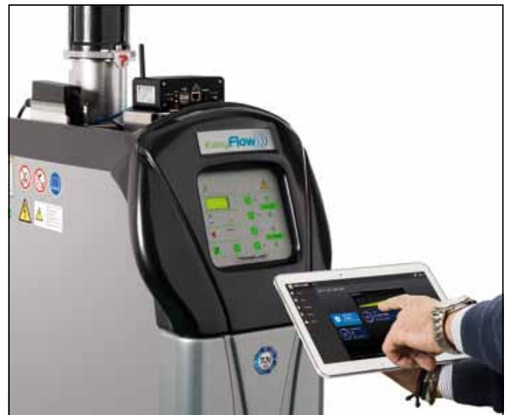
One-to-one control of the AHU via any portable device
